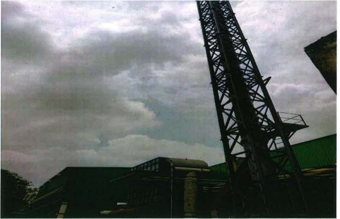
Induction Furnace Chimney and Bag filter.
