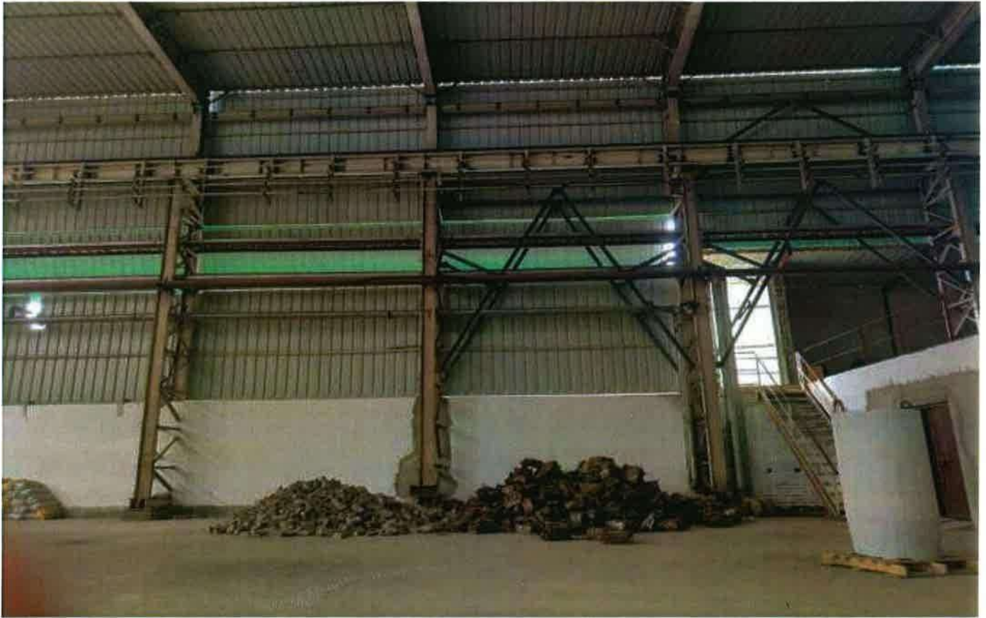
Cover Shed for raw materials.
