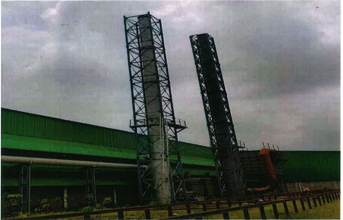
Annealing Furnace and Magnesium Converter Chimney and bag filter.
